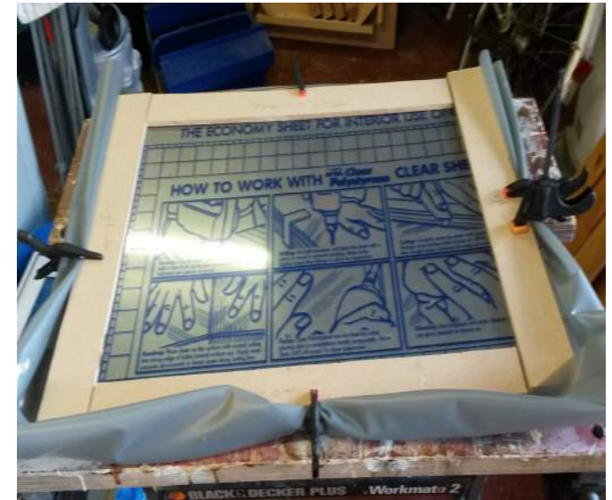
Step 15: The wooden frame with the perspex and projector material were clamped into place and screwed into place.
