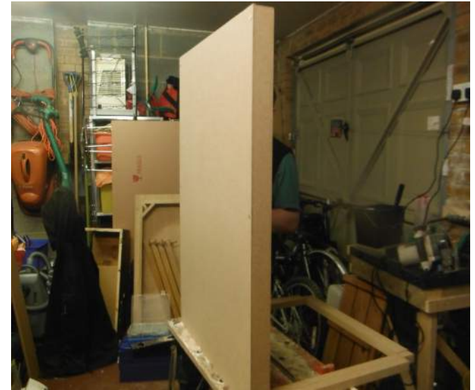
Step 3: With the frame in place the MDF panels were cut down to the right size and screwed onto the sides.
